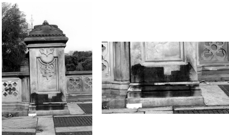
Fig. 1 Stone pillar at Bethesda Terrace, Central Park, New York, showing discoloration of a patch at the base
